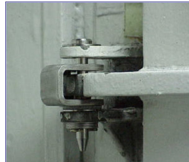
Redesigned Hinge Pins and Bushings
